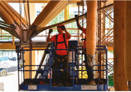
Zipper Truss Construction Image • 2016 • ©Alex Schreyer
