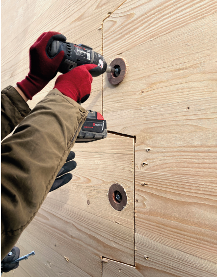
Mounting of CLT to the frame structure with cone adapters • 2023 • © t-lab
