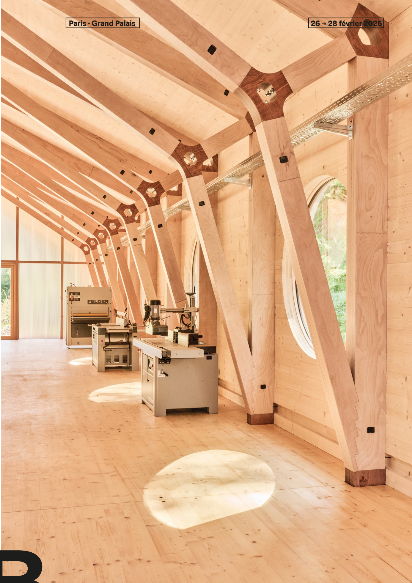
Primary structure of Educational and Research Hall for Circular Timber Construction • 2023 • ©Andreas Labes, Berlin
